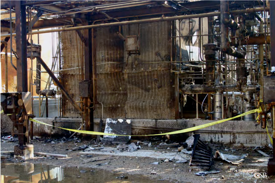
Figure 7: Explosion debris observed by CSB investigators at the base of the blast blanket surrounding the MIC tank.
