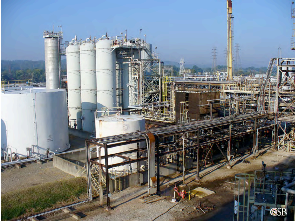
Figure 6: View of the MIC storage tank in the Methomyl/Larvin unit showing the blast blanket first installed in 1982 and then extended upward in 1994.
