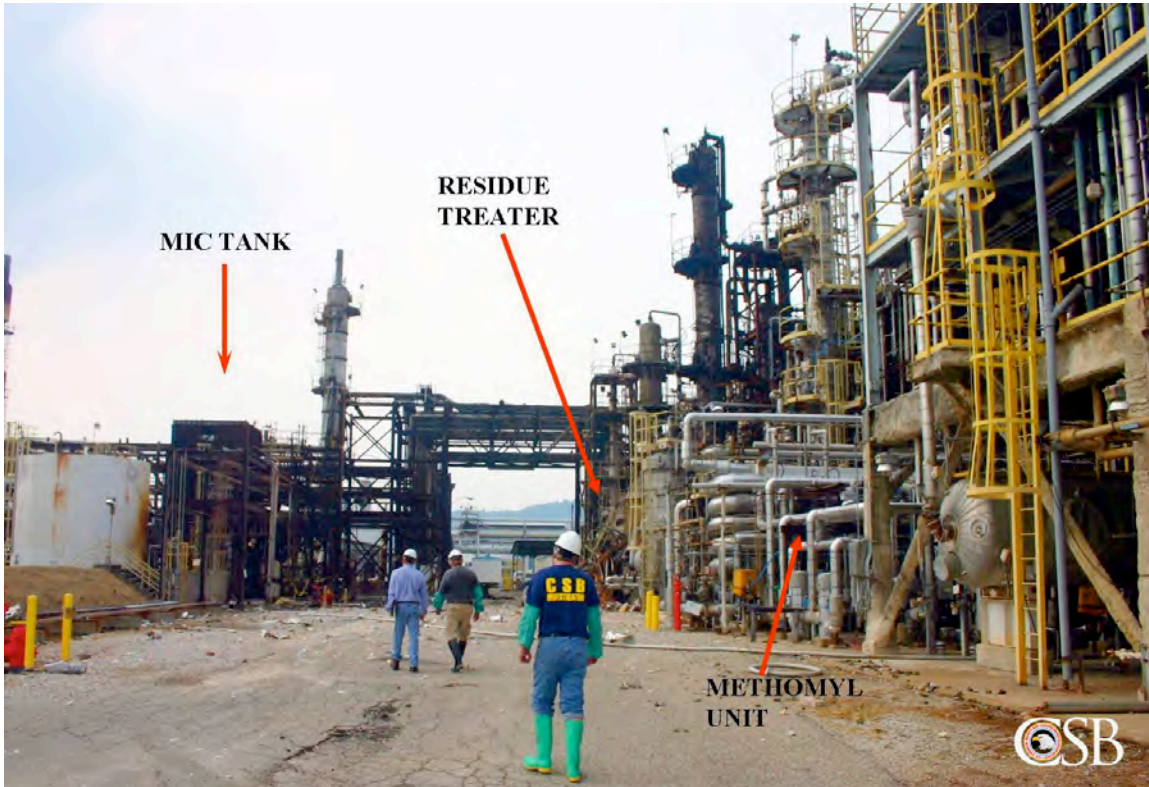
Figure 5: Ground-level view showing the proximity of the residue treater to the MIC storage tank, approximately 80 feet away across a roadway.
