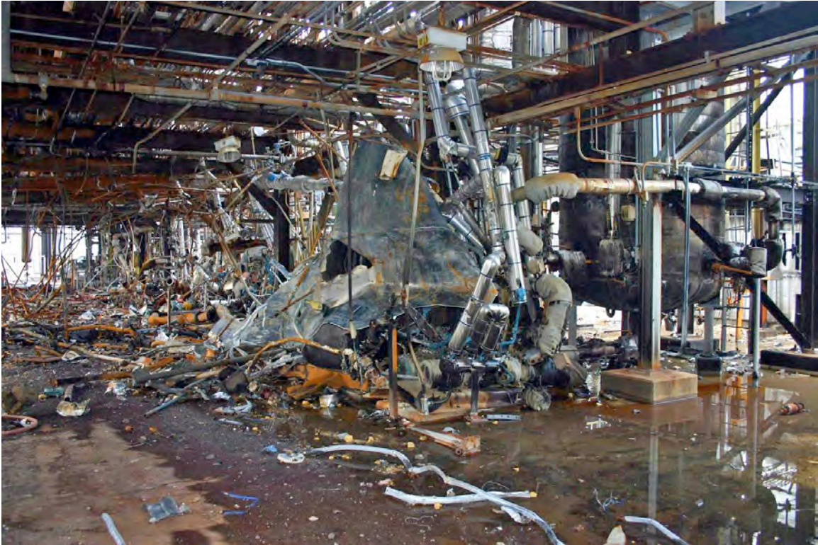
Figure 3: Equipment destruction along the trajectory of the residue treater vessel; the deformed shell of the vessel is visible at the center of the photograph.
