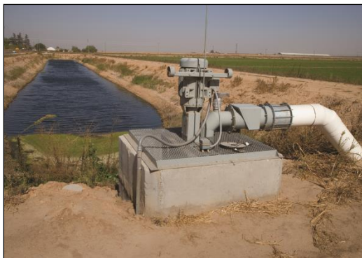
Figure 12. Tailwater Recovery and Pump
