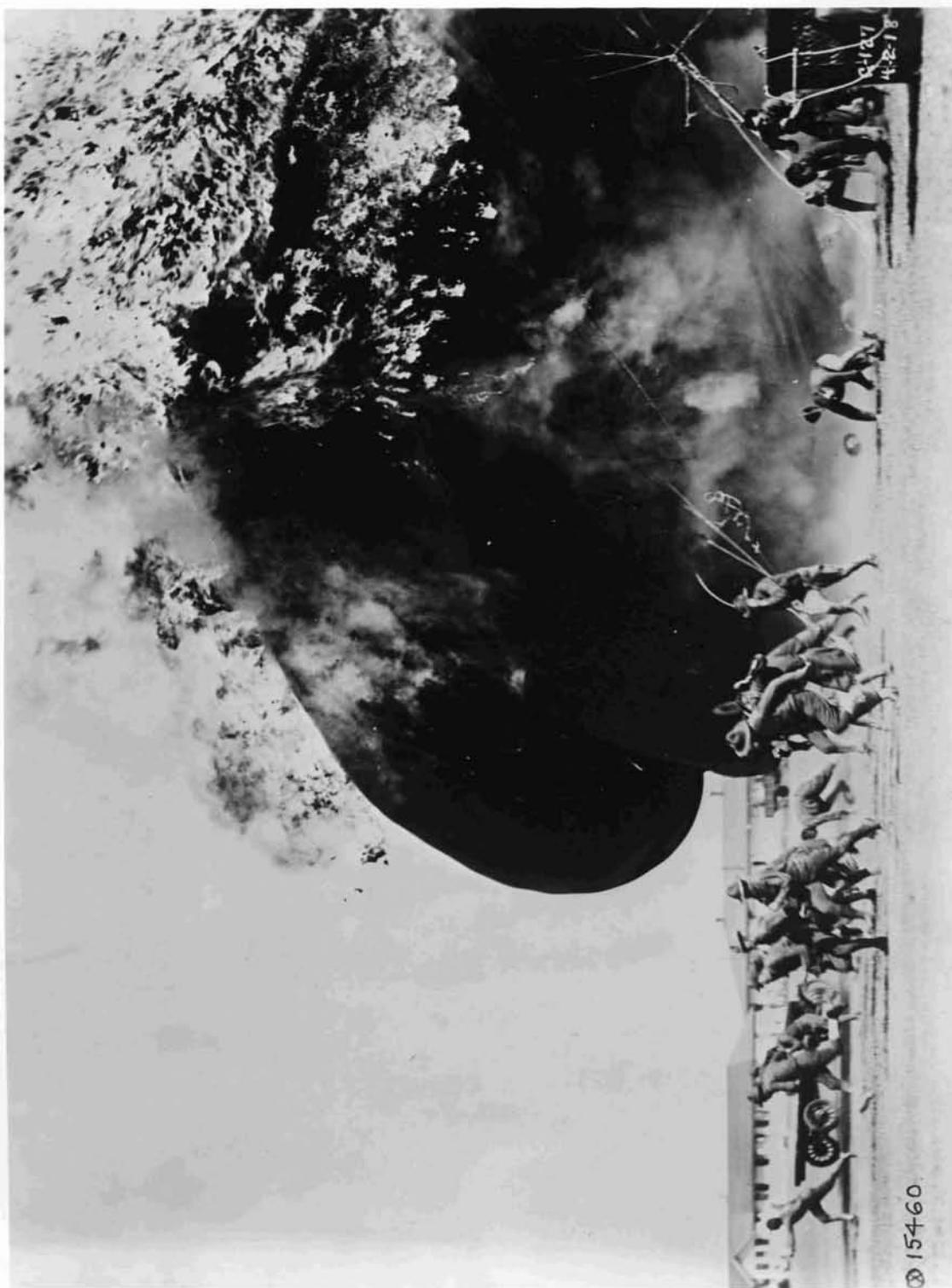
15460 - One of the most remarkable photographs of the war, - the explosion of a balloon at Fort Sill. The accident was caused in a highly exceptional manner by a static spark: the picture was withheld because it would create the impression that such accidents were common and the danger to balloonists was excessive.
