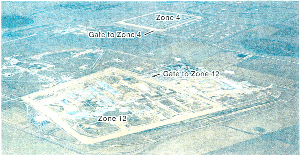
Figure 5: Aerial View of Zone 4 and Zone 12 at the Pantex Plant.
