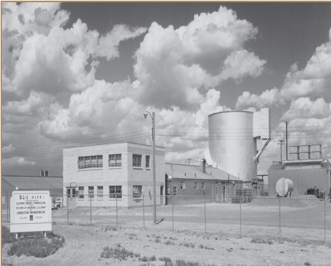
Pictured is the Stationary Low Power Plant (SL-1) at the Idaho National Engineering and Environmental Laboratory. The SL-1 was part of the Army Nuclear Power Program constructed to gain experience in boiling water reactor operations, develop performance characteristics, train military crews, and test components. The SL-1 operated from August 11, 1958, through January 3, 1961, when it was destroyed in an accident.
