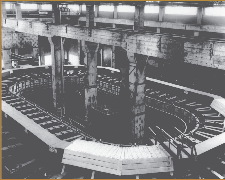
Using the electromagnetic separation process, the "alpha" calutrons at the Y-12 Plant produced enriched uranium that was fed to the "beta" calutrons for further enrichment. Pictured is the Y-12 Plant Alpha 1 racetrack.
