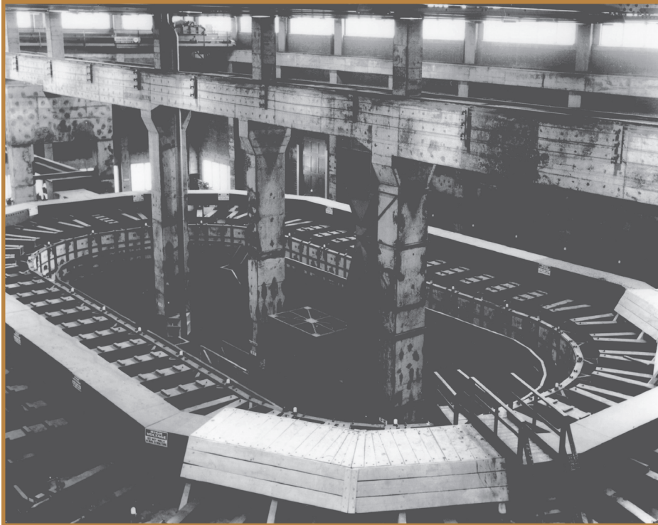
Using the electromagnetic separation process, the "alpha" calutrons at the Y-12 Plant produced enriched uranium that was fed to the "beta" calutrons for further enrichment. Pictured is the Y-12 Plant Alpha 1 racetrack.
