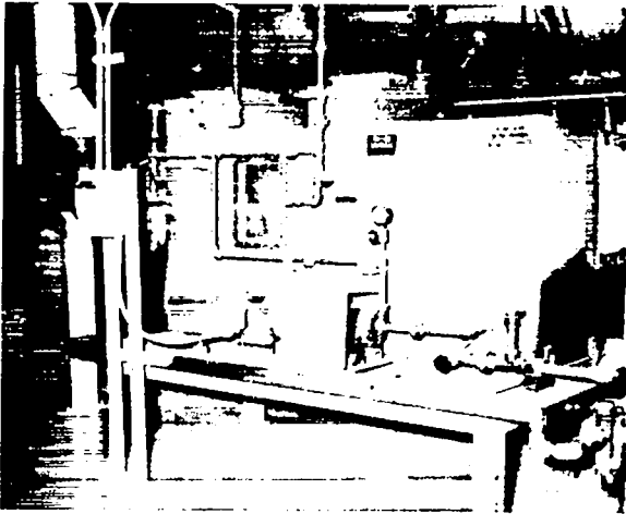
Fig. 9. Acid fume scrubber.
