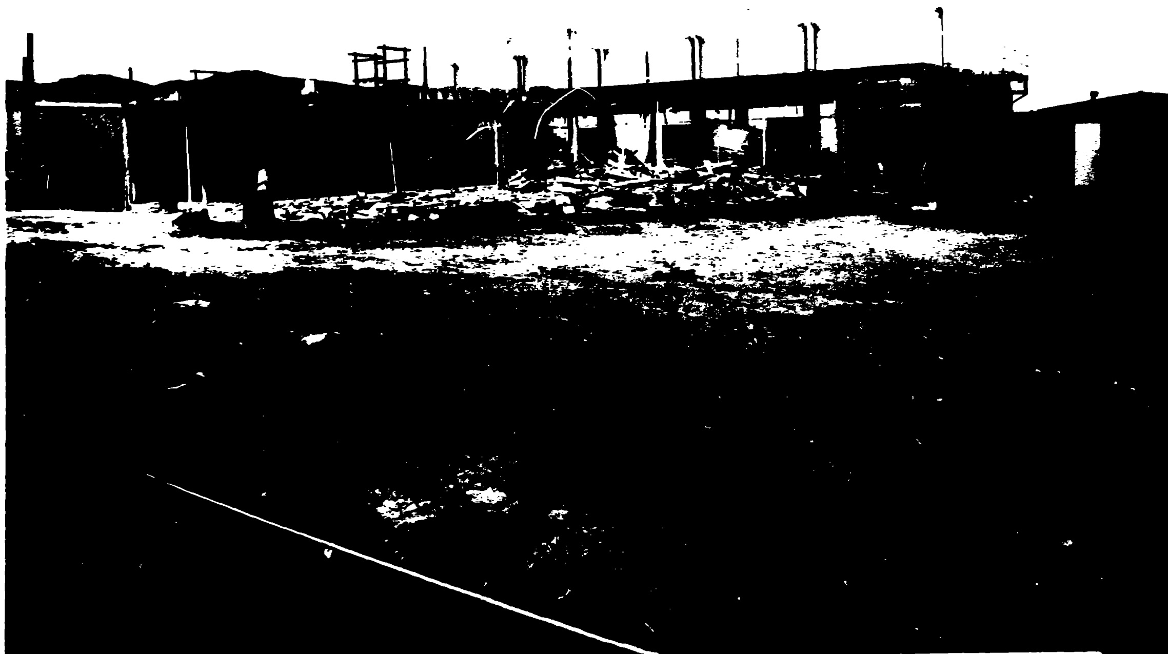
Fig. 21. INTAKE PLENUM AFTER EAST WALL HAD BEEN PULLED DOWN
