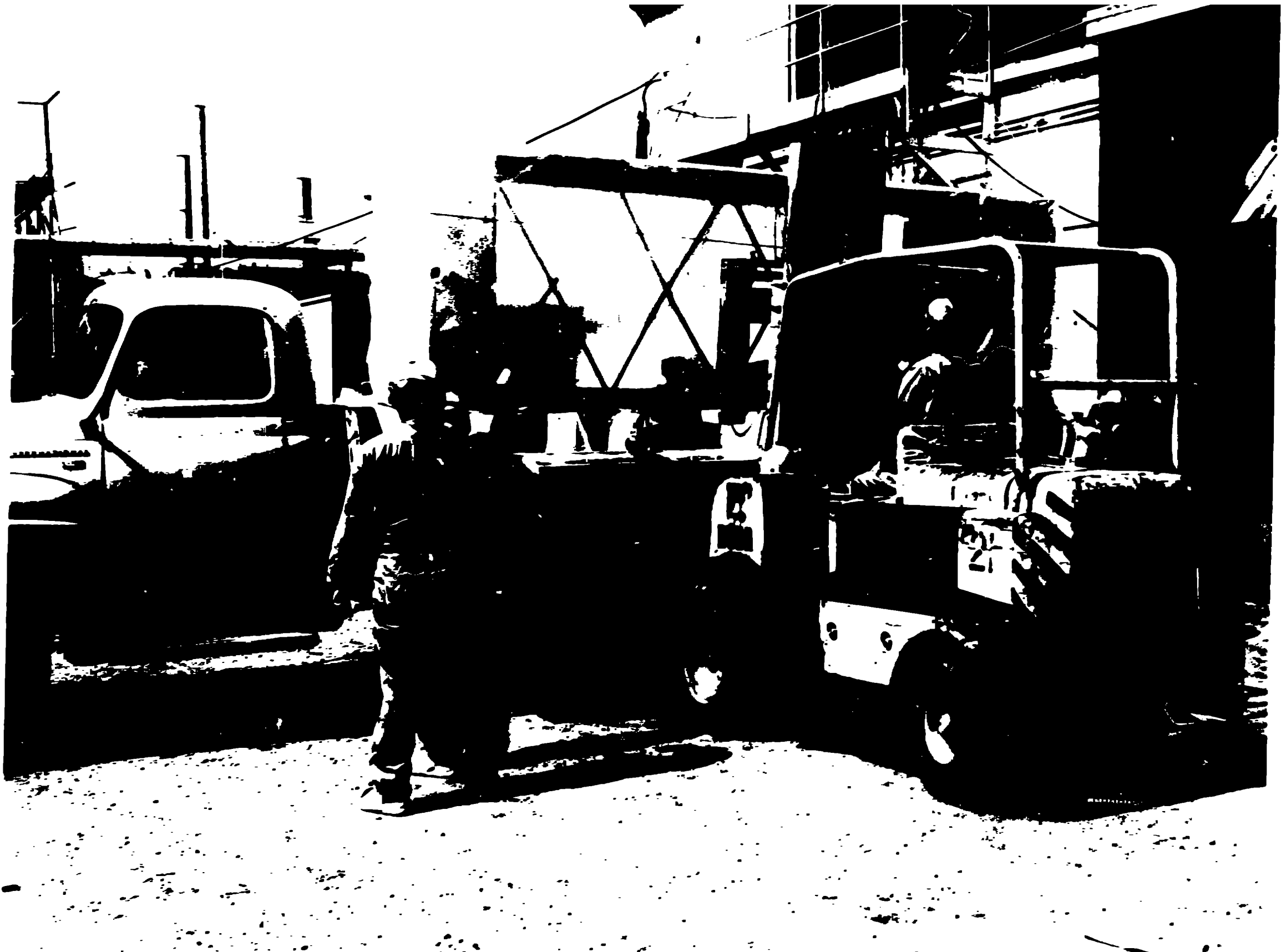
Fig. 12. PRECIPITRON FRAME READY FOR HAULING TO DISPOSAL SITE
