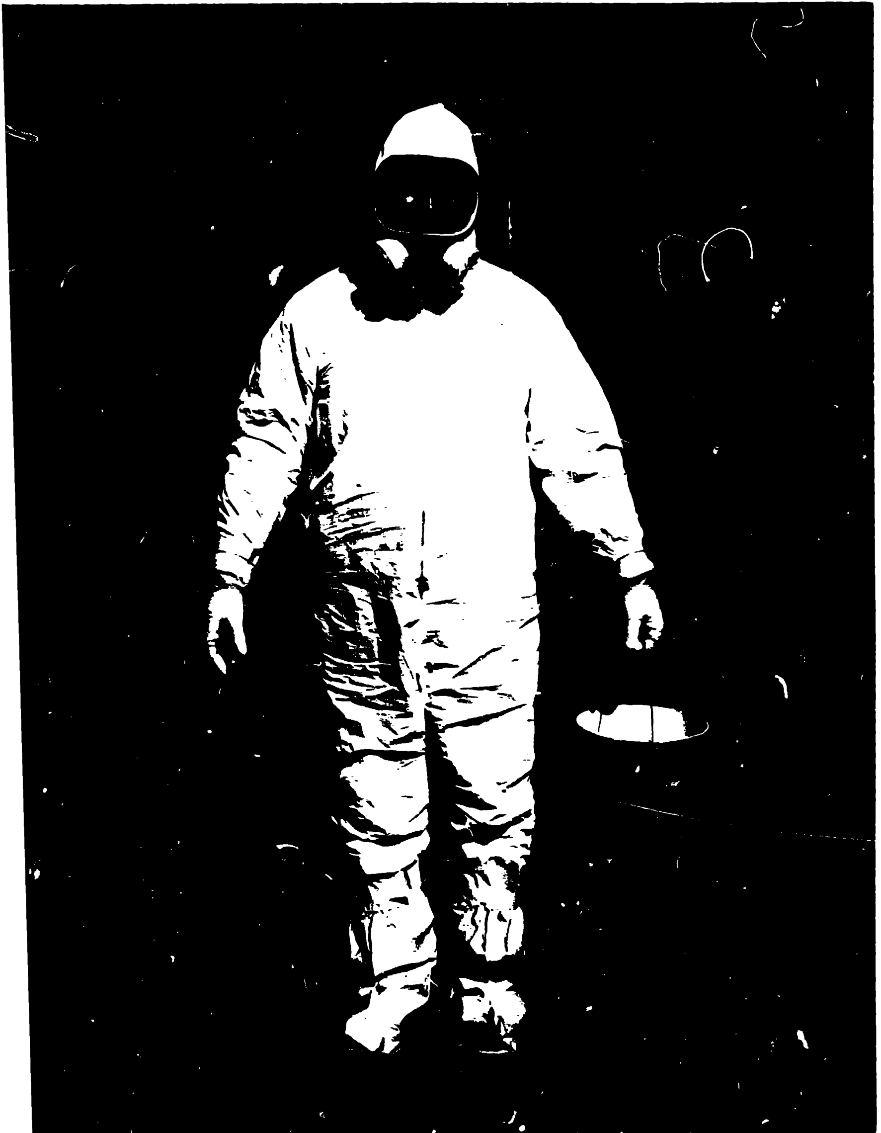
Fig. 34. WORKER SUITED UP FOR DEMOLITION WORK
