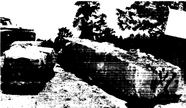
Fig. 82. Concrete-encased acid-sewer lateral after removal from H Building (the concrete was found intact).
