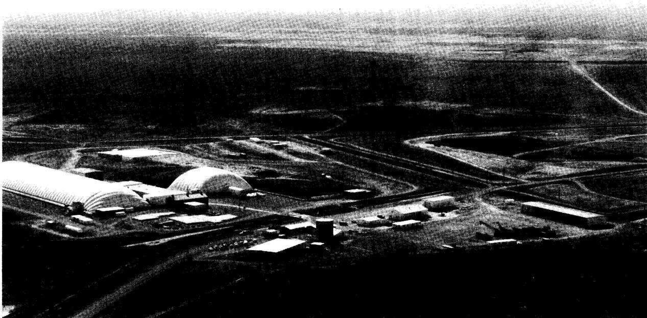
Photo credit: U.S. Department of Energy
