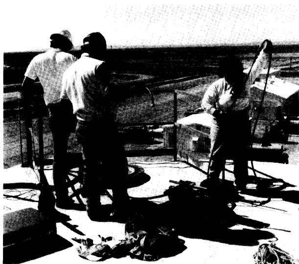
Photo credit: U.S. Department of Energy
