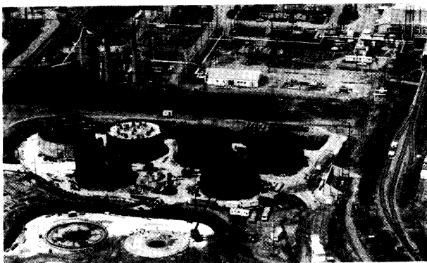
Photo credit: U.S. Department of Energy
