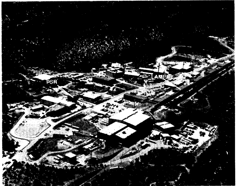
This aerial view of Technical Area 53 shows the proton linear accelerator of the Los Alamos Meson Physics Facility, which produces high-intensity pulses of protons for research in medium-energy physics; the Proton Storage Ring, which converts some of the LAMPF pulses into higher-intensity proton pulses; and LANSCE, where those proton pulses are used to create high-intensity pulses of neutrons for research in materials science.
