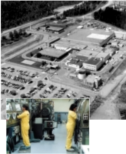
The plutonium facility at Los Alamos is developing the capability to remanufacture small lots of plutonium pits and now carries out all surveillance activities necessary for stockpile stewardship. All experiments and tests are conducted inside a glove-box environment (inset).
