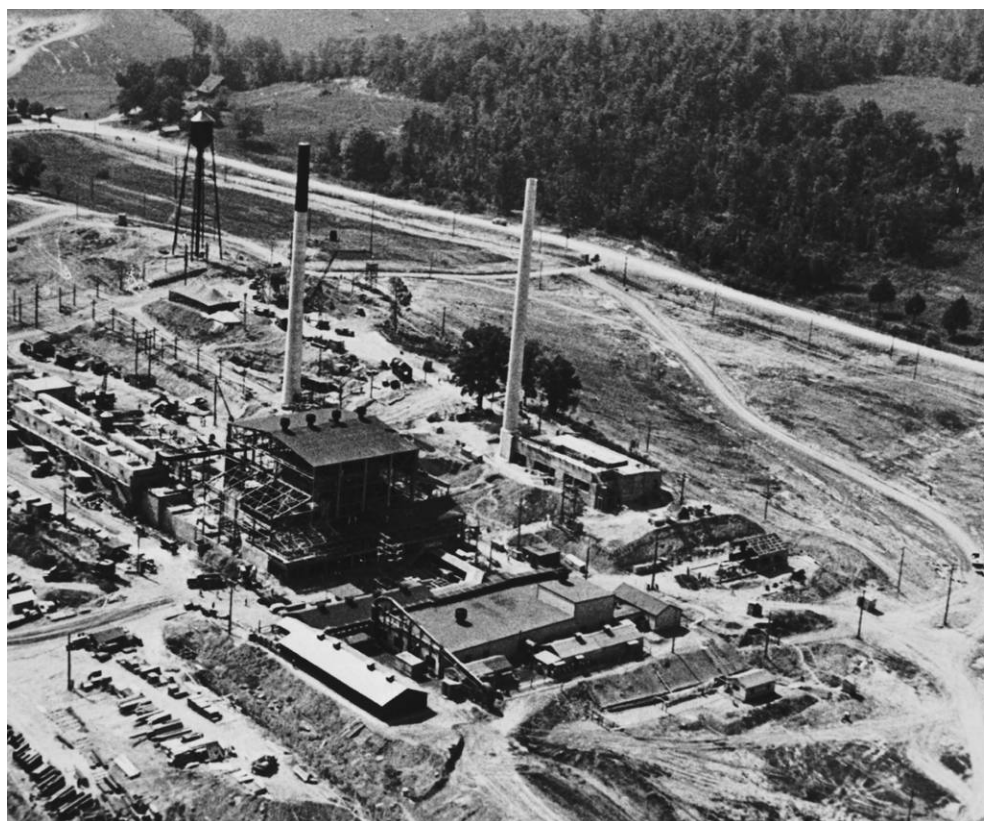
Fig. 3. The Graphite Reactor and the concrete cells of the chemical processing pilot plant under construction in August 1943. (ORNL History Photo 152)
