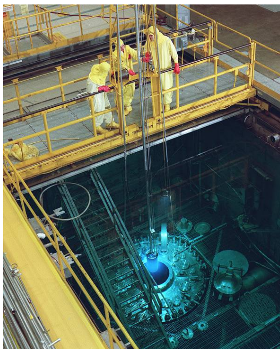
Fig. 51. Replacement of HFIR fuel element. (ORNL Photo 11299-92)
